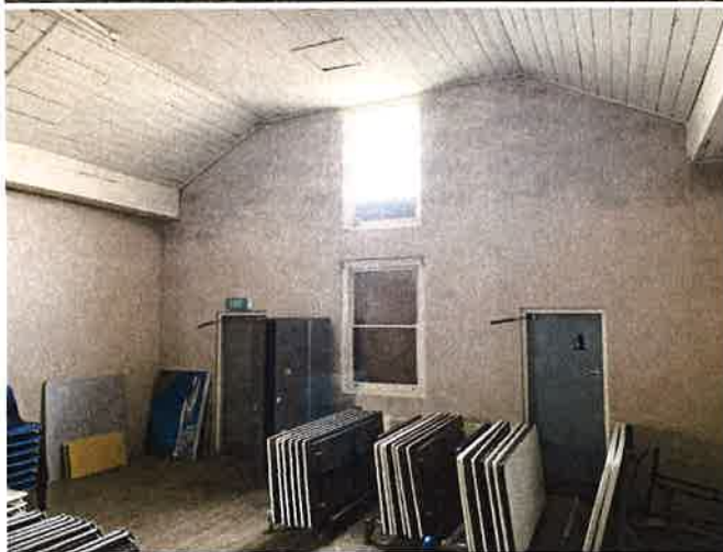
Figure 17 Signs of falling damp. Courtesy architects King + Campbell.
